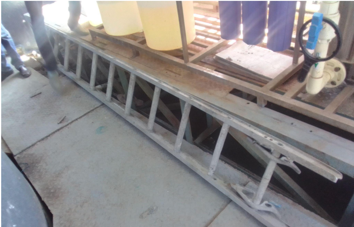
The narrow access to the tank and the ladder used to go inside the 10-ft Tank
